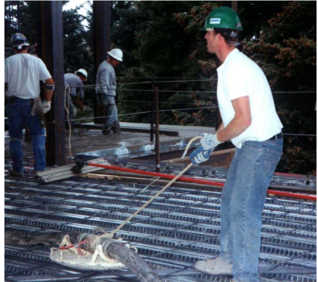
Fig. 1. Laborer pulling concrete-filled hose secured to skid plate.
